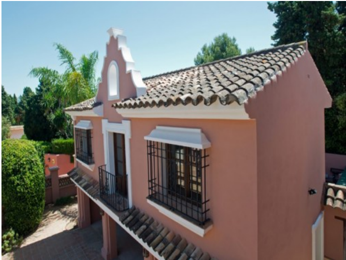
House views with balcony
