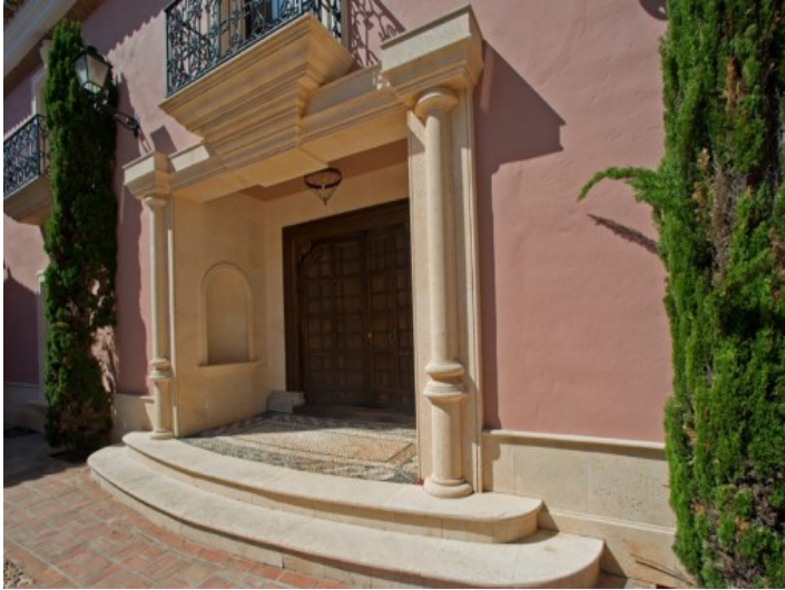
Main entrance with wooden door
